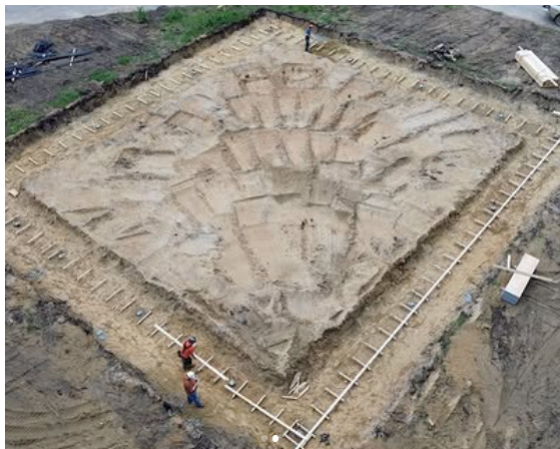
Thanks to RNF Ventures Ltd., for the aerial views of the gym construction.
